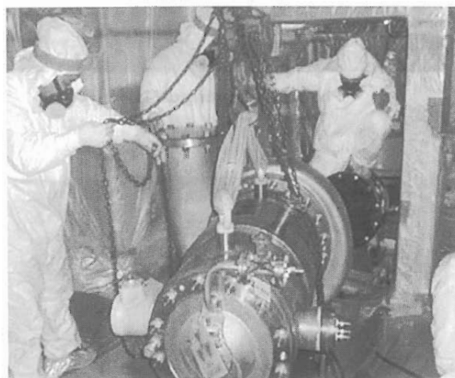
Photo 4 Dismantling of Main Pump
