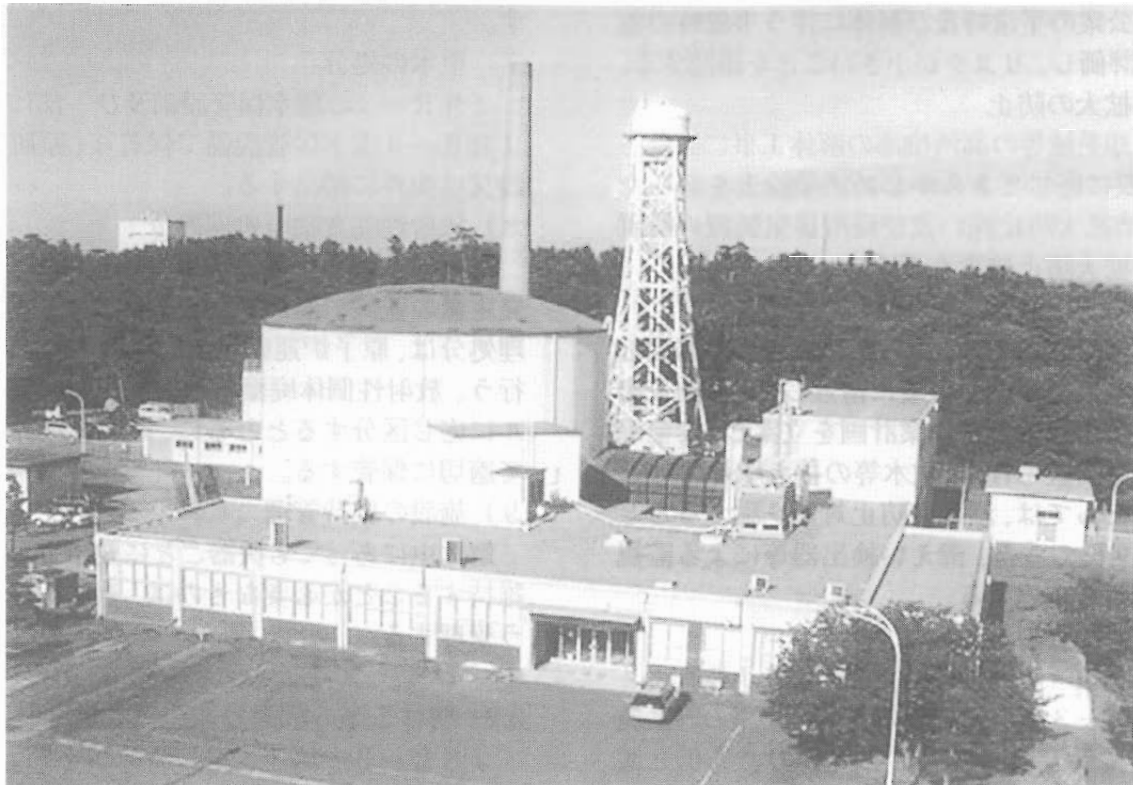
Photo 1 Overview of JRR-2
