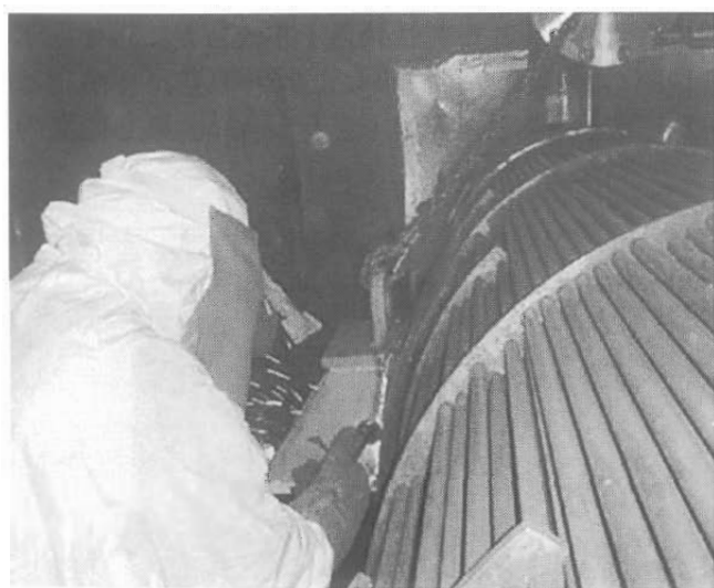
Photo 3 Dismantling of Heat Exchanger
