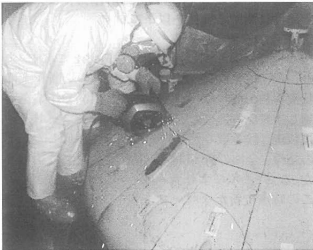
Fig.16 The Conditions of the Cutting Work
